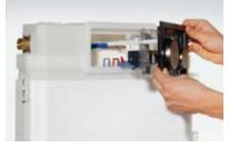
For servicing, the entire engineering unit, including the lever mechanism, cover and push plate, can be removed. **All settings are therefore retained.**
