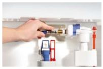
After the shell construction: The reinforced pipe is attached to the push fittings system on the filling valve with no need for tools.
